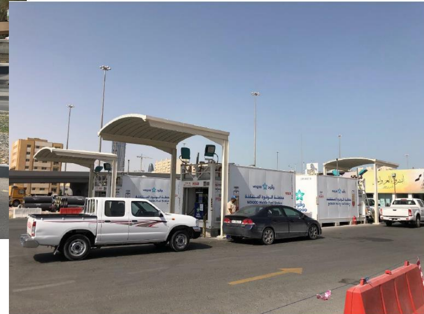
Wogod Service Station, Qatar
